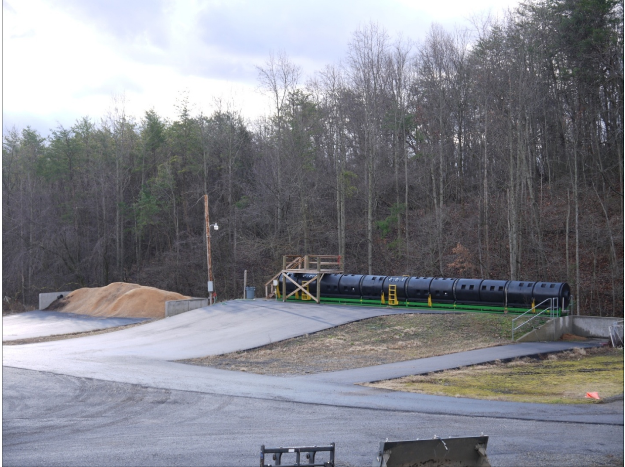
Figure 1. Rotary Drum System. There is a loading platform above the first door, and a second door is located near the center of the drum.
