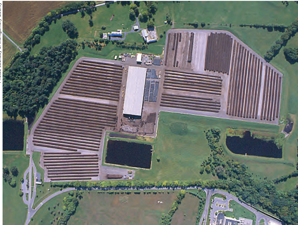
The Montgomery County yard trimmings composting facility sits on a 48-acre asphalt pad. After curing, compost is moved under an 80,000 square foot pavilion (center), where it is allowed to fully mature.
